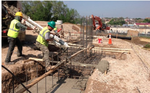
Foundation work for the new addition at Frederick Elementary School in west Baltimore
